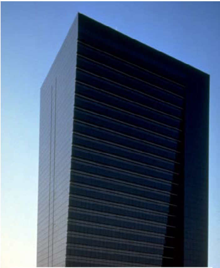
GEORGIA POWER - Corporate headquarters of the Georgia Power Company, acquired by build-sale-leaseback. The company's prior commitment for purchase by a financial institution provided the basis for construction financing. All design and project management aspects were under the direction of George T. Heery, FAIA RIBA FCMAA, at the time Chairman of Heery International.
